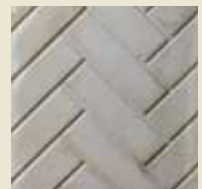
Interior Firebrick Refractory Herringbone
